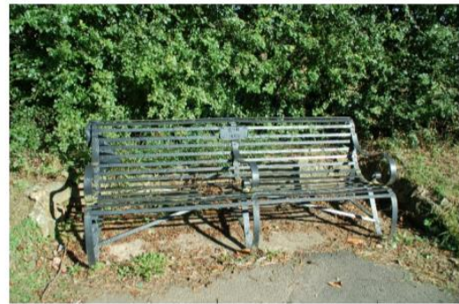
Wright's Lane-good condition, light clean reqd.
