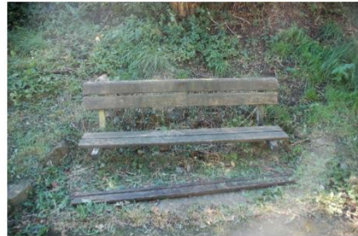
Meadows Rise-repair doubtful, replacement reqd?.
