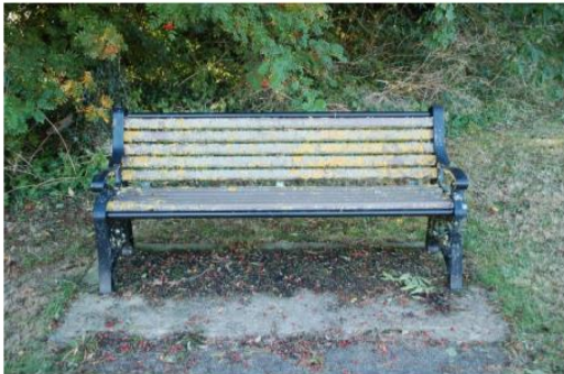
Rookery Lane-good condition, needs cleaning
